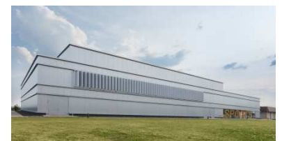
Neubau Physical Fitness Center, Katterbach
